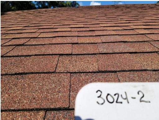
3024-2 Asphalt Shingle Typical Exterior Roof
